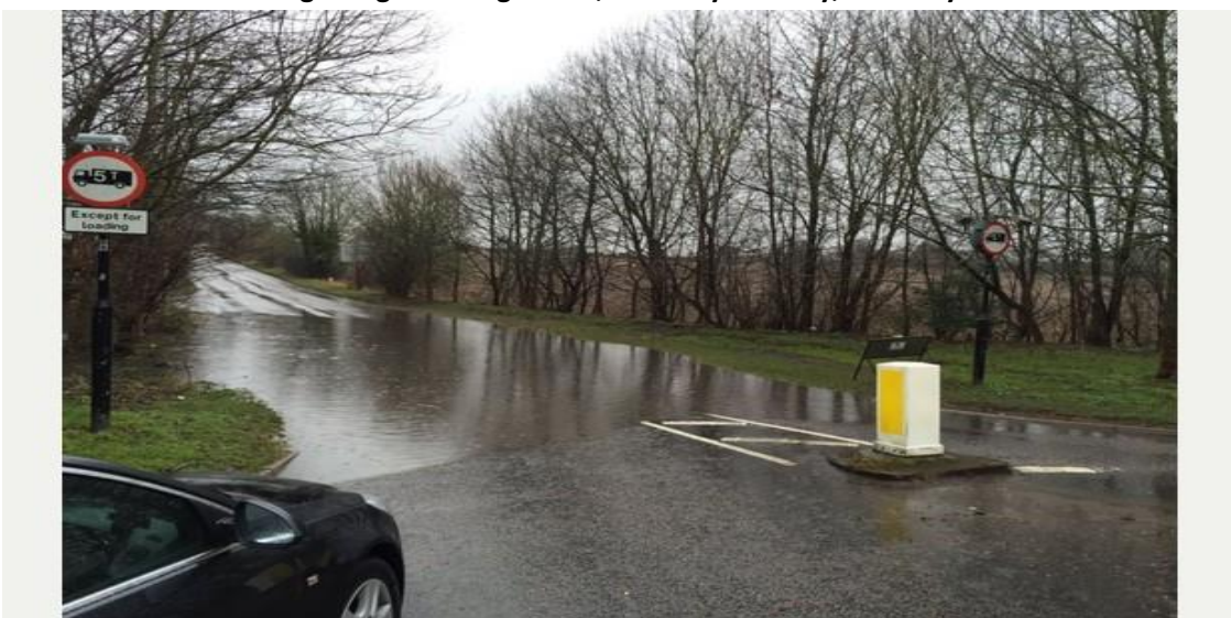
Little Wymondley Flooding, 9 March 2016 - Arch Road/Stevenage Road Junction
